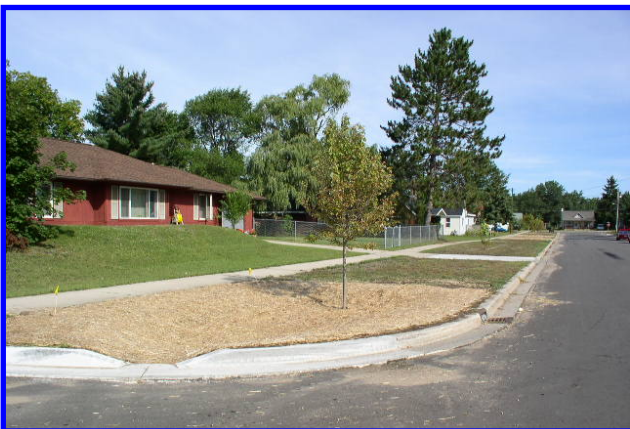
One of 86 rain gardens recently created in Phase I of the Grayling Stormwater Project. Note the curb used to allow water to enter the basin.
