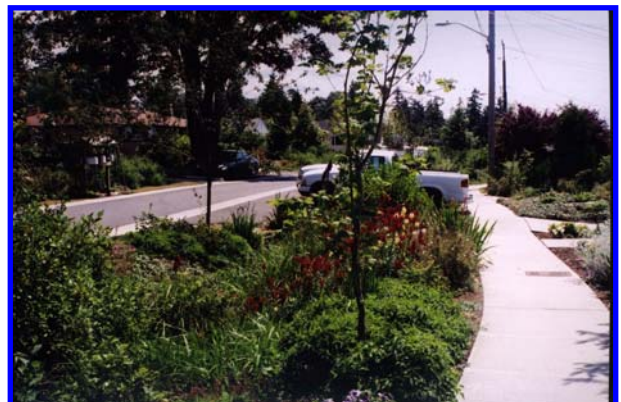
The shallow depression area in the rain garden above is hard to observe because of the lush plant growth that has occurred. This basin in the street right-of-way above is from a project in Seattle similar in concept to the Grayling project.
